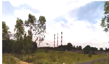
Figure 4- Bakreshwar Thermal Power Project across agricultural fields
