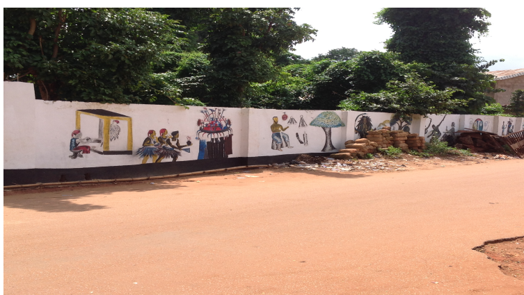
Plate 5: A section of the perimeter fence
