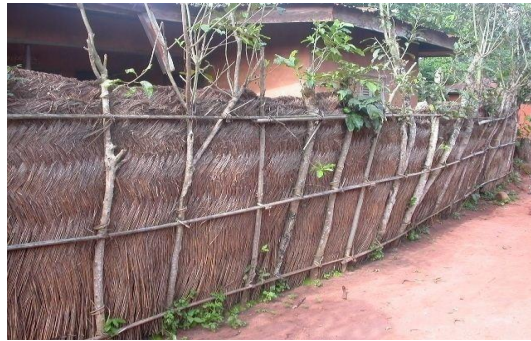
Plate 2: Traditional fencing ( uho ) constructed with ogbu ( Ficus spp ) and azana ( Hyparrhenia spp )
