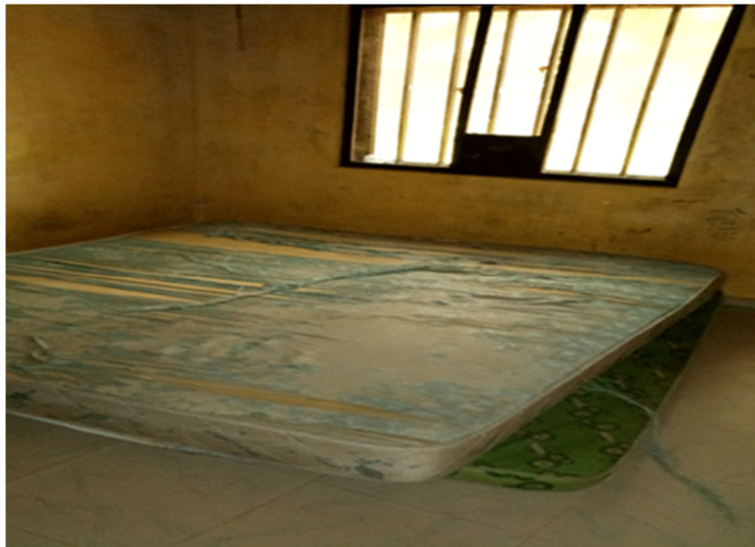
Plate 3: Showing inner view of a student hostel in Okomu National Park. Source: Field Survey, 2018
