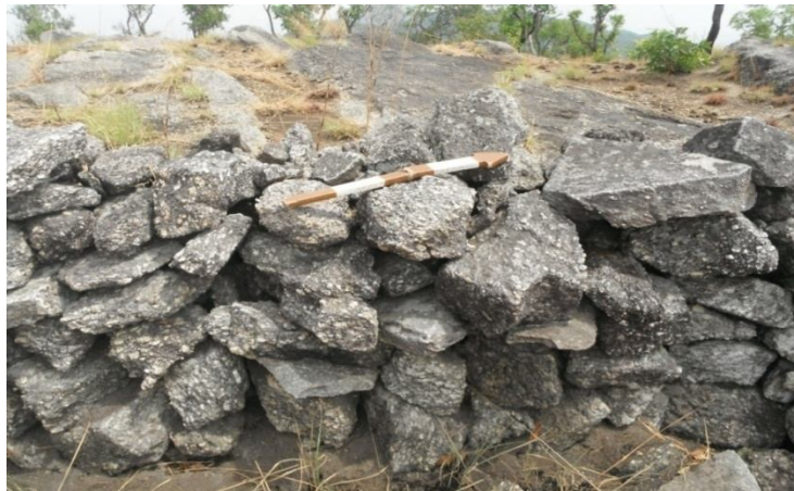
Figure 8: Part of a Dry Stone Wall on Gbanger Hilltop Abandoned Settlement.
