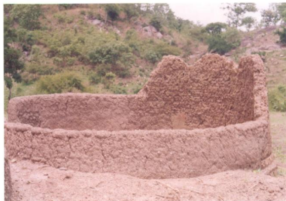
A section of Bernard Fagg's house under reconstruction.
